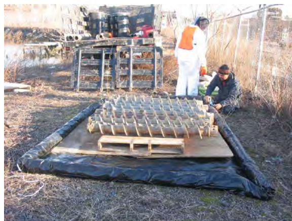
Photo 4: Decontamination pad setup along eastern boundary of the Site.
