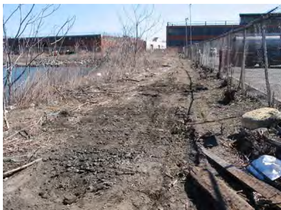
Photo 15: Graded the disturbed areas along the eastern shoreline of BCI.
