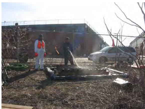
Photo 5: Crew used a garden hose connected to a fire hydrant to clean the augers.
